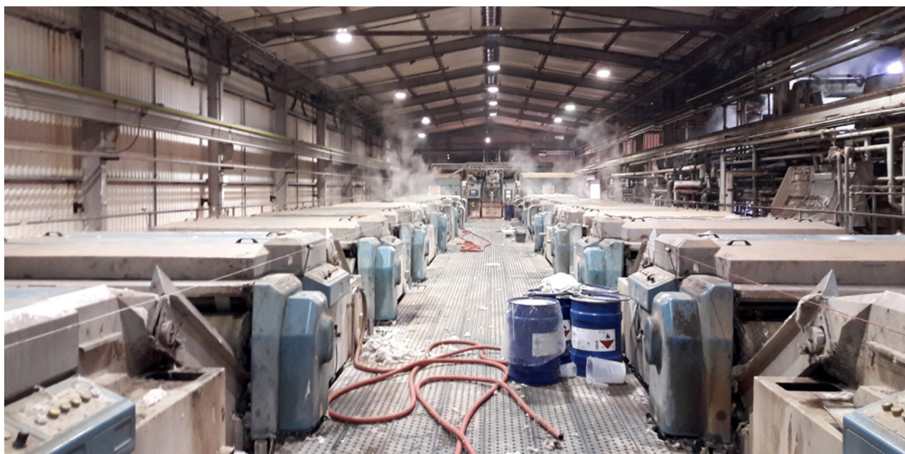
Photo 2. Scouring line in Bradford, UK in 2017. Photo by A. Matsin
