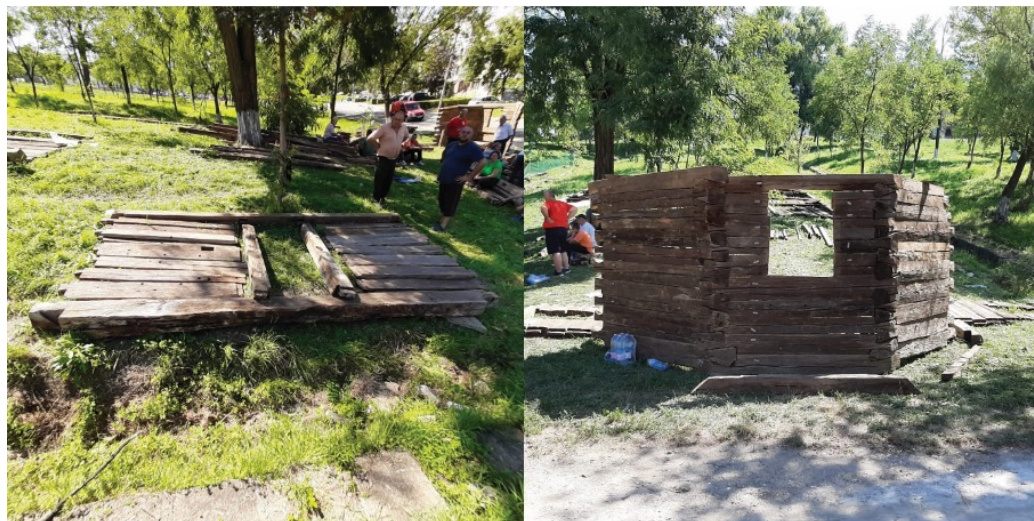
Figure 6. Wall mock-up phase, before final assembly
