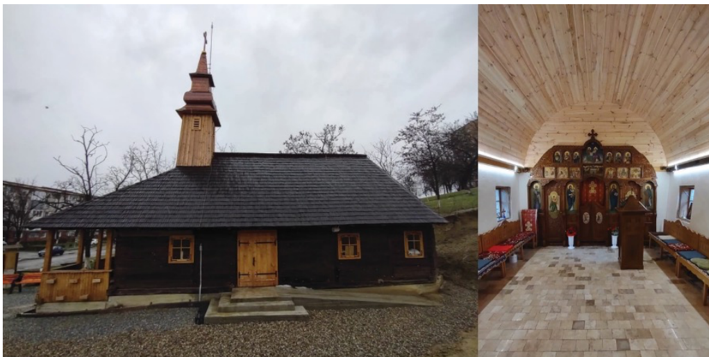
Figure 8. Pictures showing the exterior and interior of the finalized work
