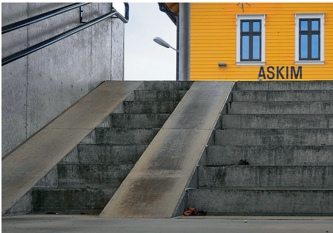
Figure 2.6. Specially designed ramp
