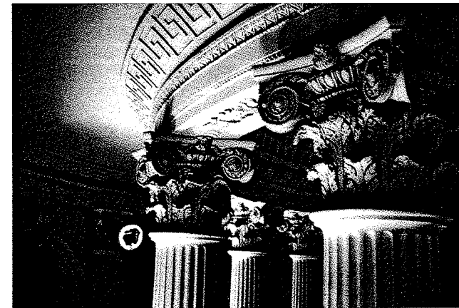
St Andrew's Kirk showing the annular arch supporting the dome. The carved Corinthian capitals are exceptionally sophisticated.
