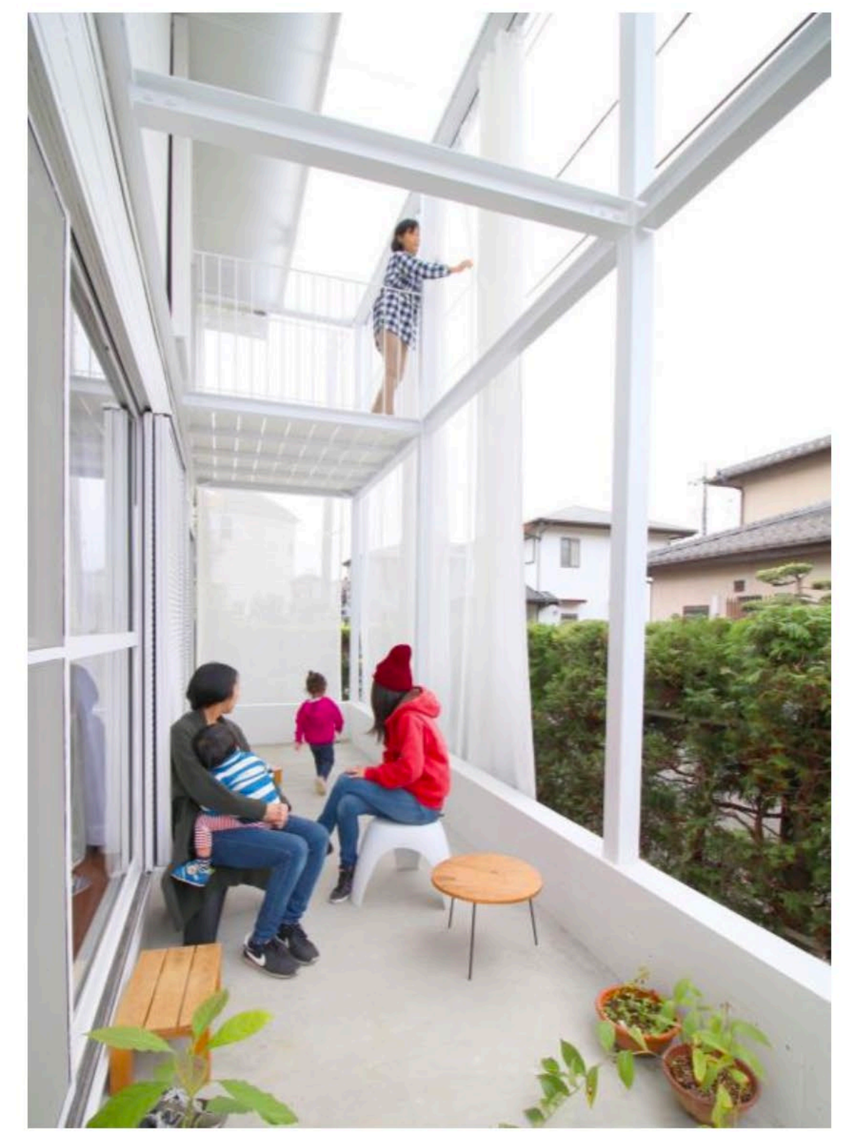
Typical example of independent exterior building structure
