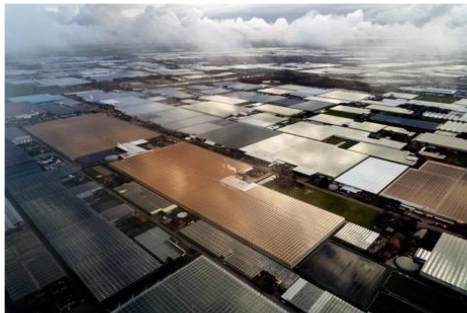
Westland, Netherlands https://www.thecivilengineer.org/
