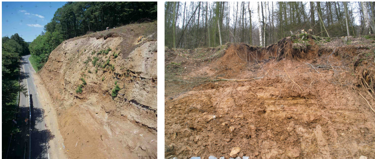
Figure 1a/b: Characteristic landslides in Quaternary hillslope sediments in the southern Solling area.
