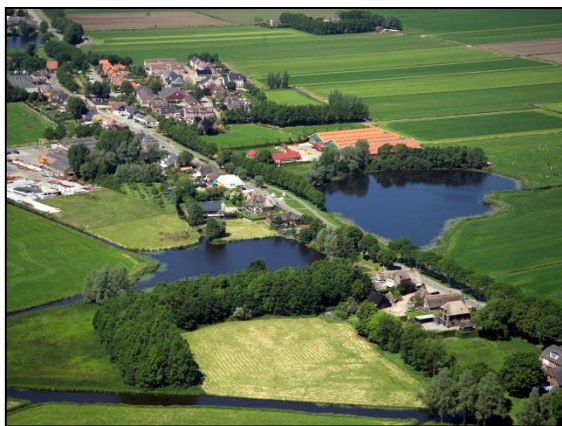
Dike breach scars Former storms Zuiderzee Kamperzeedijk
